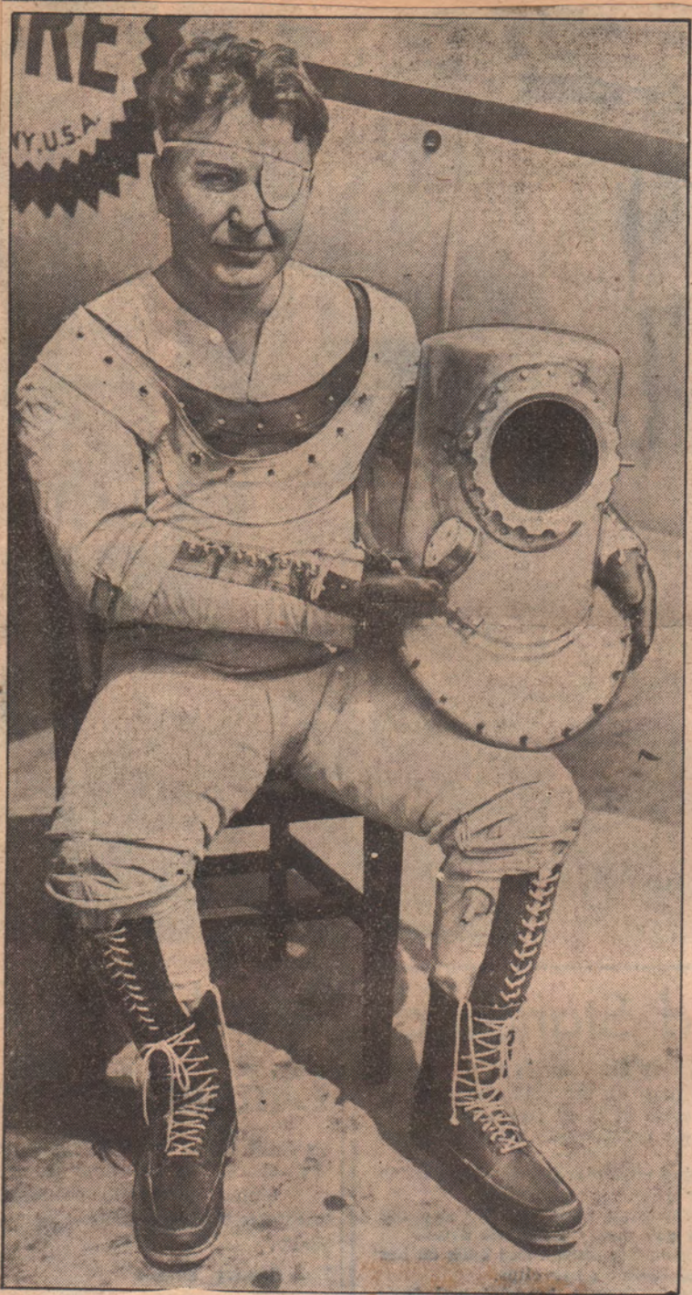
READY FOR STRATOSPHERE —Here is the stratosphere suit of Wiley Post, noted round-the-world flyer. Post was photographed in the suit in Chicago. Left is a closeup of the fur-lined outfit with aluminum helmet. Above is a demonstration of how oxygen is pumped into the tank that goes with the ensemble. (AP)
